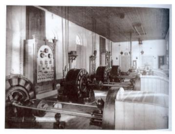
First 3-phase transmission system installed in Sweden between Hellsjön and Grängesberg 1893 voltage 9650 V, 70 Hz, 70 kW
