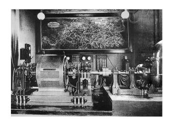
170 kW transferred 175 km from Lauffen hydropower station to the exhibition area at 13000-14700 V
